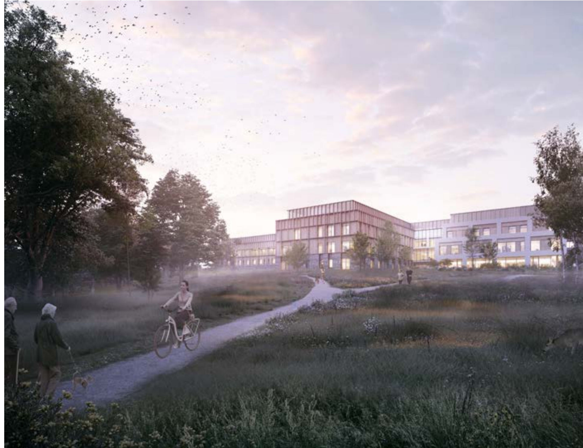
View to the facility from the Taff Trail cycle path Golygfa i'r cyfeuster o lwybr beicio Taith Taf
