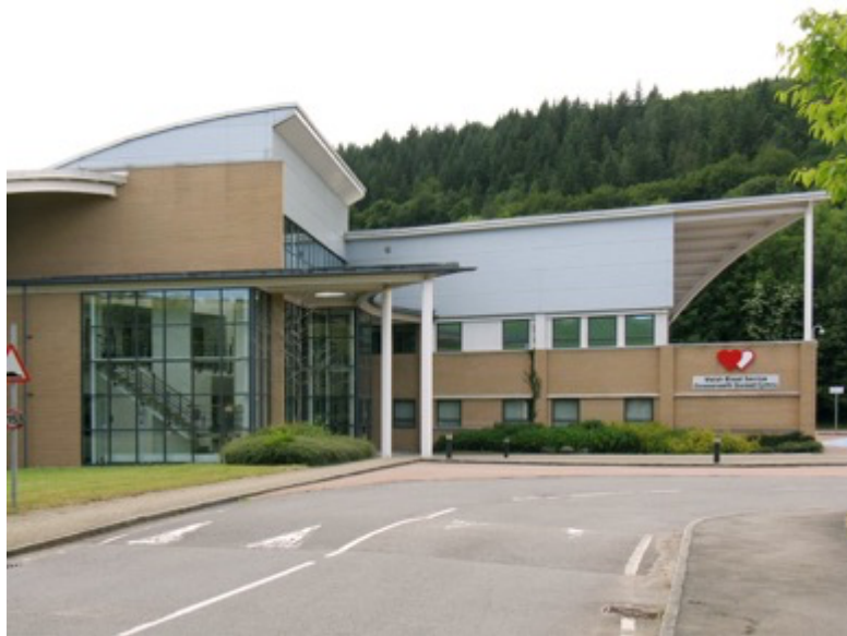
Figure 8: Existing Main Entrance
